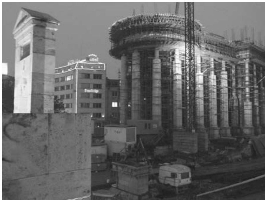
New construction, Skopje
